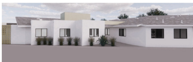
Lynwood facility under construction
